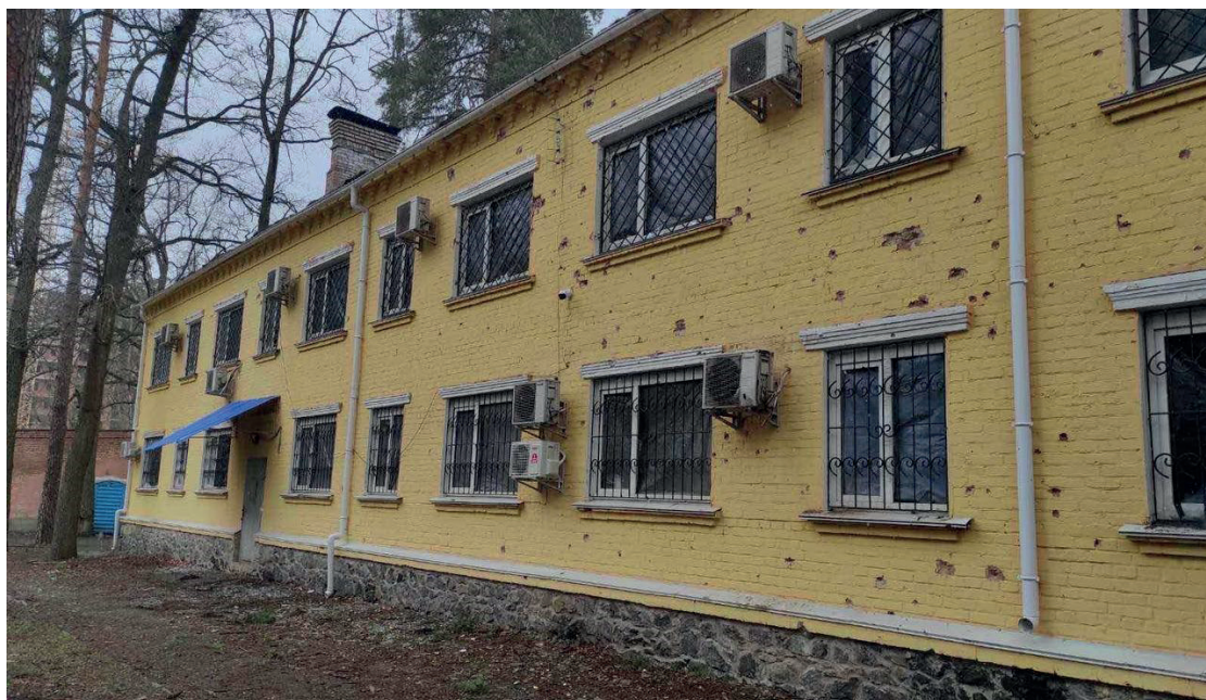
The building of the Irpin City Court of the Kyiv Region after the occupation
