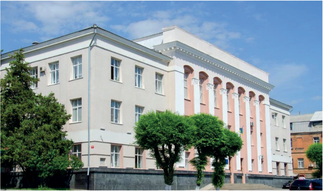
The building of the Vinnytsia Court of Appeal
