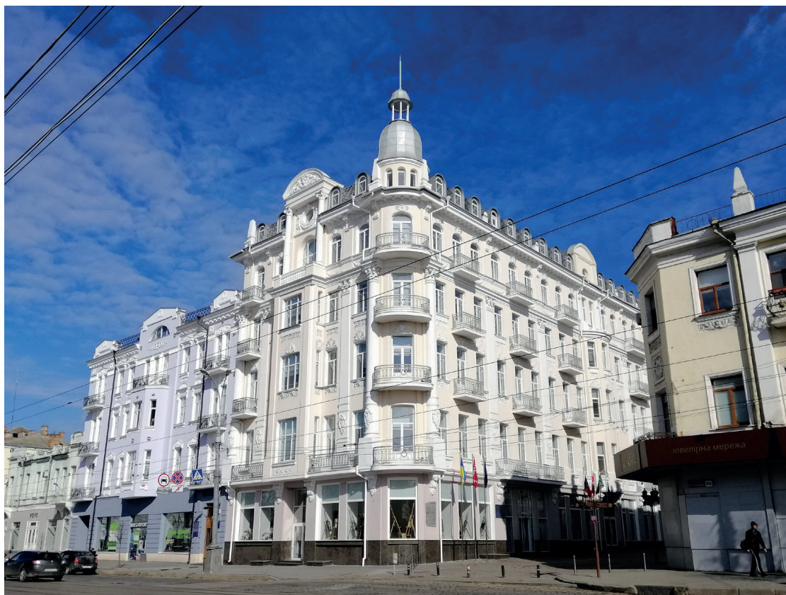
The building of the Seventh Administrative Court of Appeal in Vinnytsia
